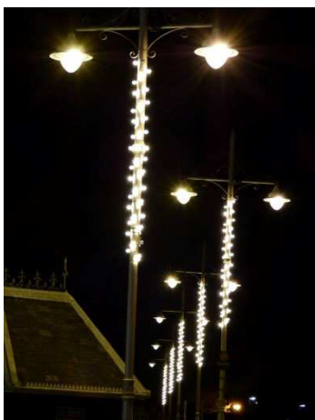
Replacement lighting in Waterloo Square
